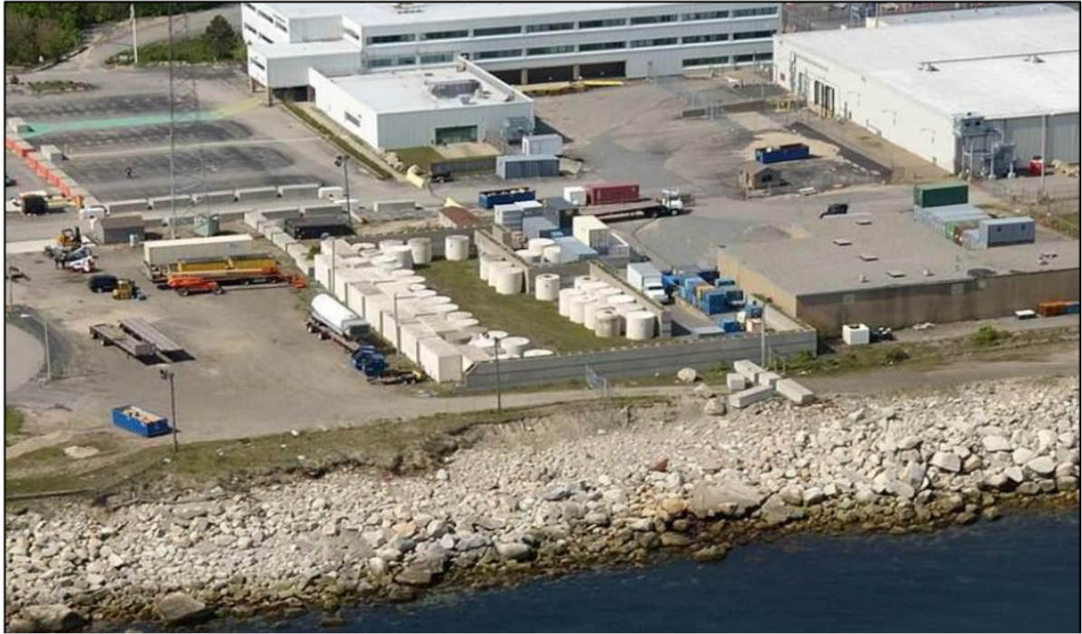
Figure 8. The white containers pictured here are LLRW containers, located about 30 ft. away from Cape Cod Bay. At least one of these holds radioactive waste and many more will likely be filled during decommissioning. Also shown to the right of the storage area is the LLRW building containing equipment that compresses materials to be stored for shipment.
